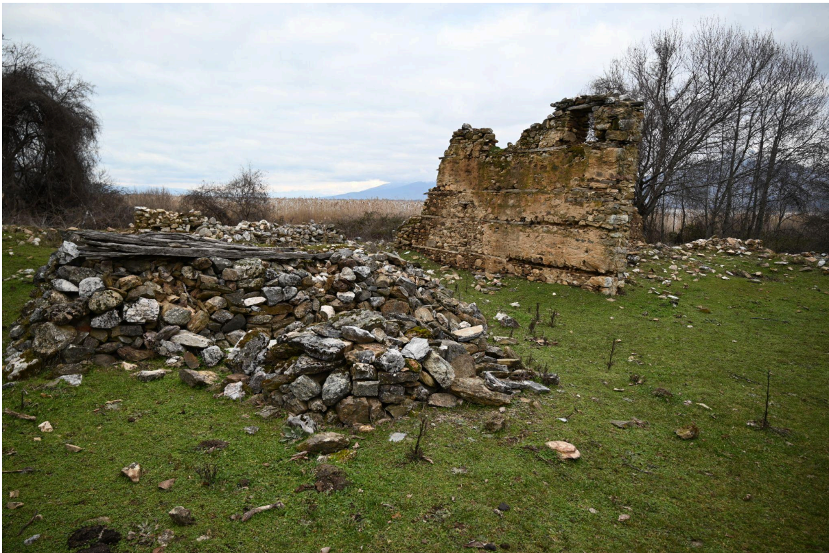
This location functions as a terminus within the route. From here, visitors must descend and follow an alternative path leading toward the next installation site. © TRIETHNES FESTIVAL
